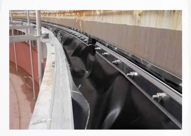
We can adapt any seal design to suit your particular roof configuration.In particular if you have tanks that suffer from tank shell distortion we can tailor make a sealing system that will provide an effective sealing solution. We offer the following types of tank seal.
