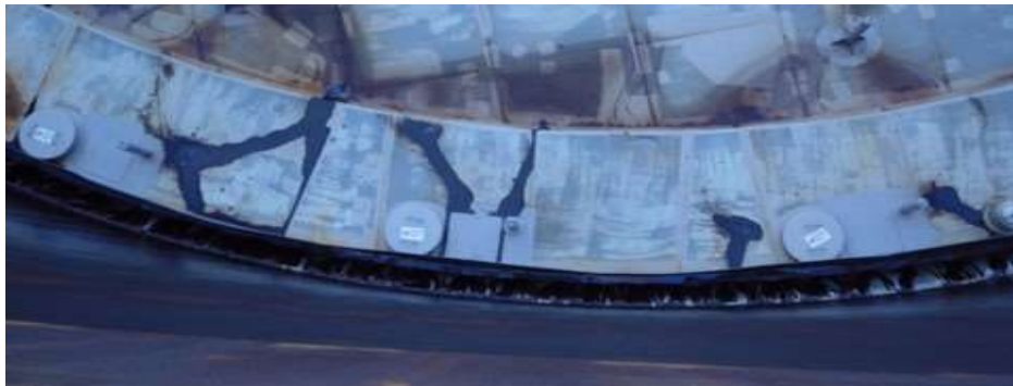
Floating Roof crude collection
