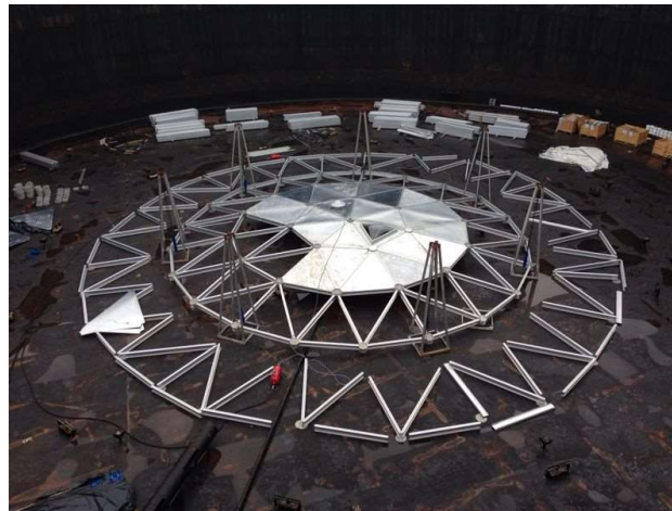
Alu Geodesic Dome Roofs
