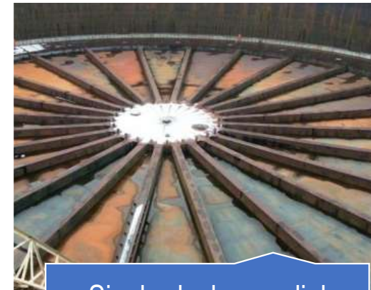
Single-deck w. radial beam stiffeners (SIPM)
