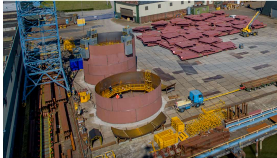
External Floating Roofs
