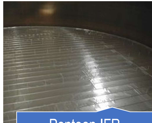
Pontoon IFR Deck Sheeting
