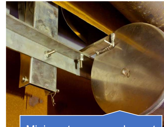
Mini-pontoons complement existing buoyancy
