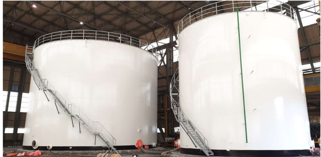
External Floating Roofs
