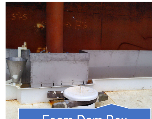
Foam Dam Box around Gauge Pole
