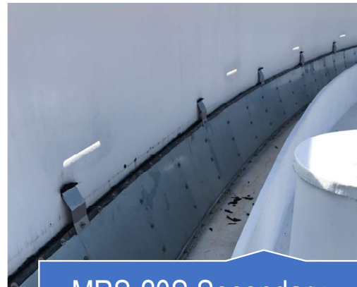
MRS-20S Secondary Compression Plate Seal
