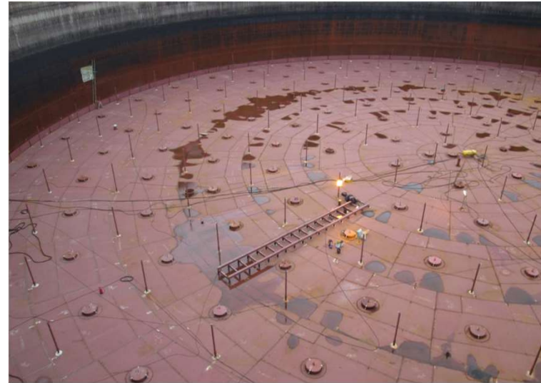
External Floating Roofs
